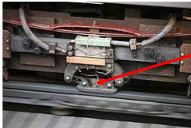
Train Collector Shoe "rubbing" 3 rd rail
