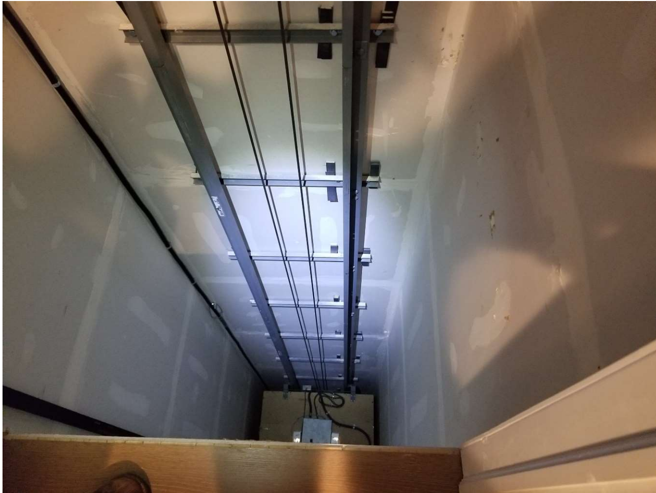
Four Floor Elevator Shaft
